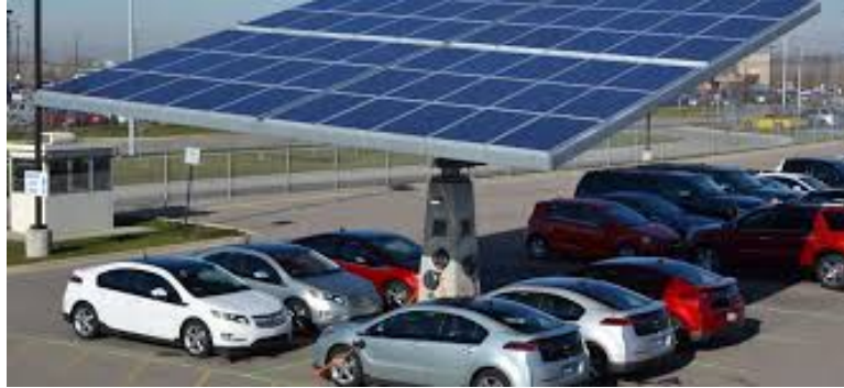
Figure 1: Electric/Hybrid vehicles charging while parked
