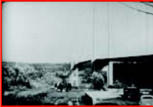
Figures 5a: Tacoma Narrows Bridge
