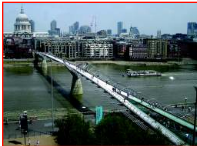
Figure 6: The Millennium Bridge
